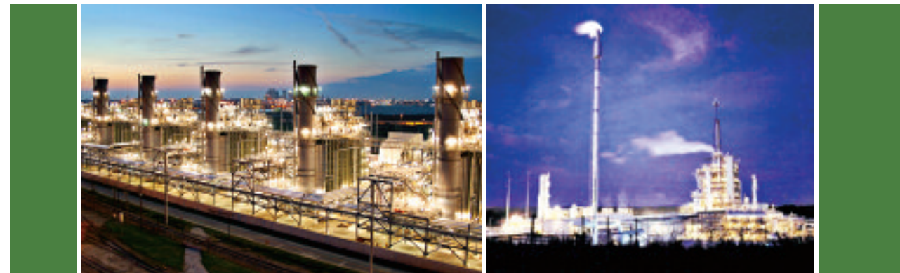
▲ Tampa Electric’s Polk Power Station
